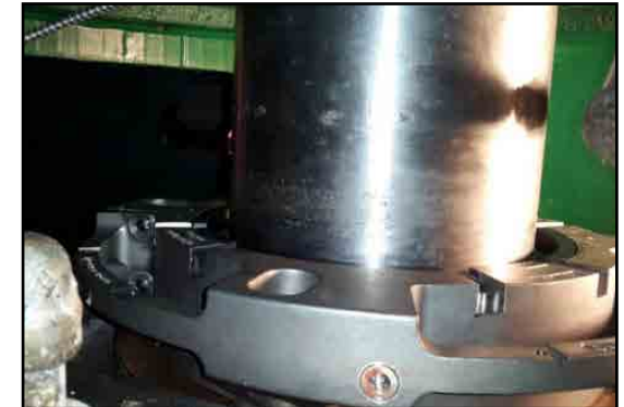
Vertical pump installed with 442.
