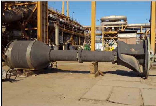
Brine vertical pump being serviced for repairs.
